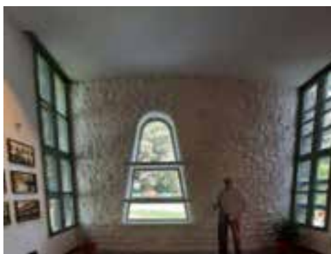
Figure 2.29: The final restored wall Source: Author
