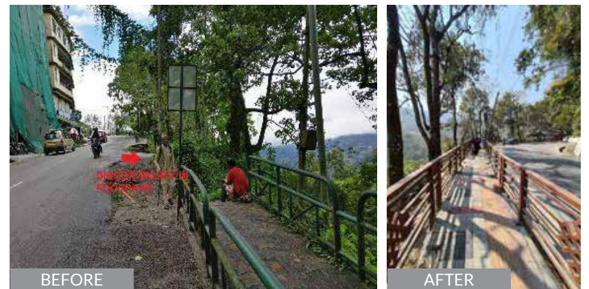
Figure 15: Old footpath surface & railings (Left) & new footpath surface & railings (Right) Source: DPR, 2018 (left) & IIT Kharagpur Survey (right)
