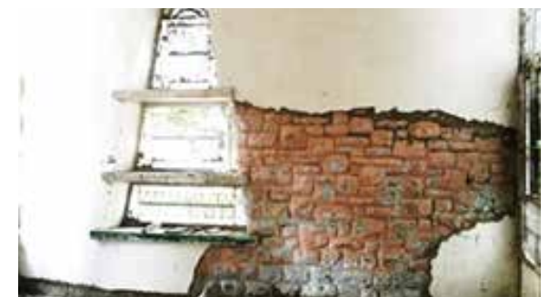
Figure 2.28: Plaster chiselled out to reveal original rubble masonry wall Source: Ar. Deepika Gandhi
