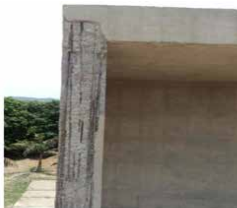
Figure 2.22: Image of the Open Hand monument before restoration Source: CSCL
