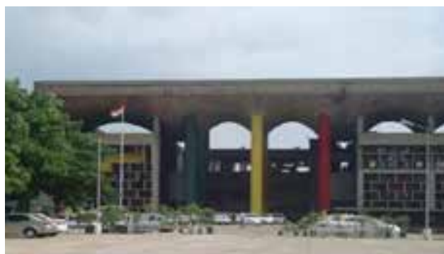
Figure 2.4: Plaza used for parking in front of High Court Source: Chandigarh Heritage Report by Heritage Conservation Committee of Chandigarh
