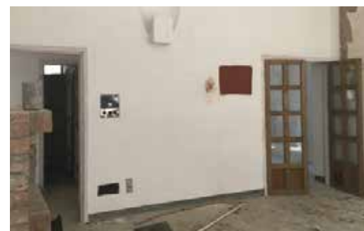
Figure 2.27: The final restored light niche; Source: Author
