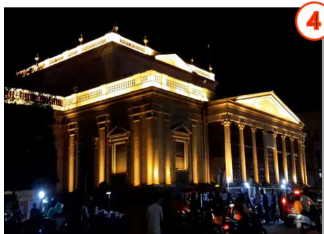
Figure 6 shows the faced lighting of Government Post Office (Source: primary)
