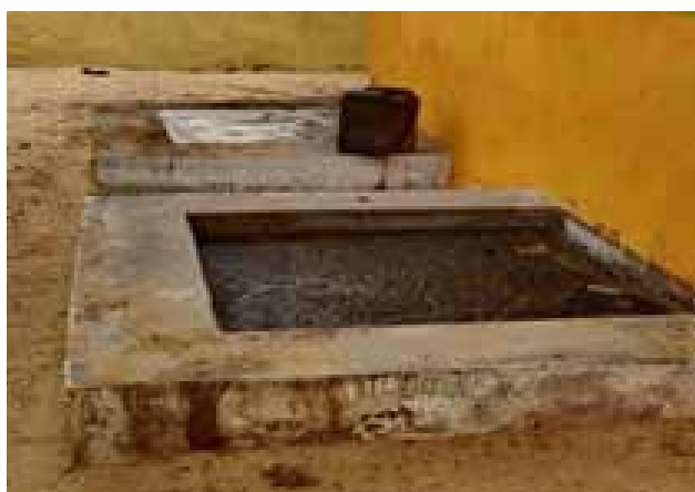
Figure 12. Leachate pit adjacent to the compost tub Source: Author
