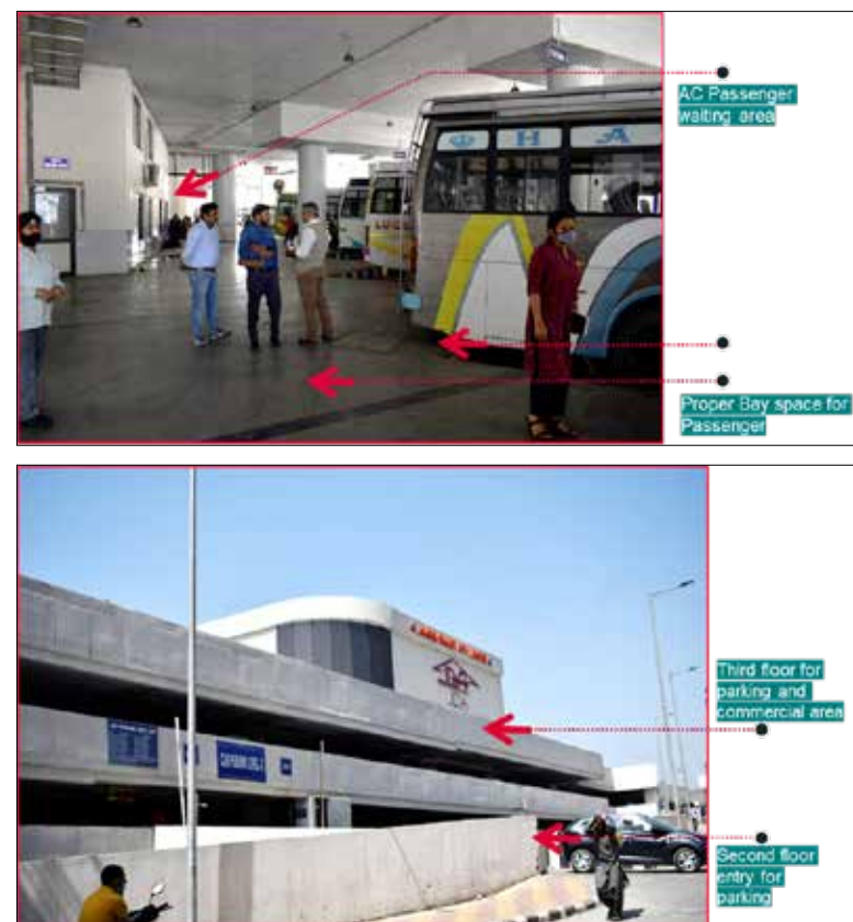
Figure 3.6: Bus stand facility
