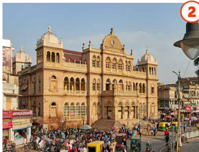
Figure 4 shows the façade restoration of Town Hall (Source: primary)
