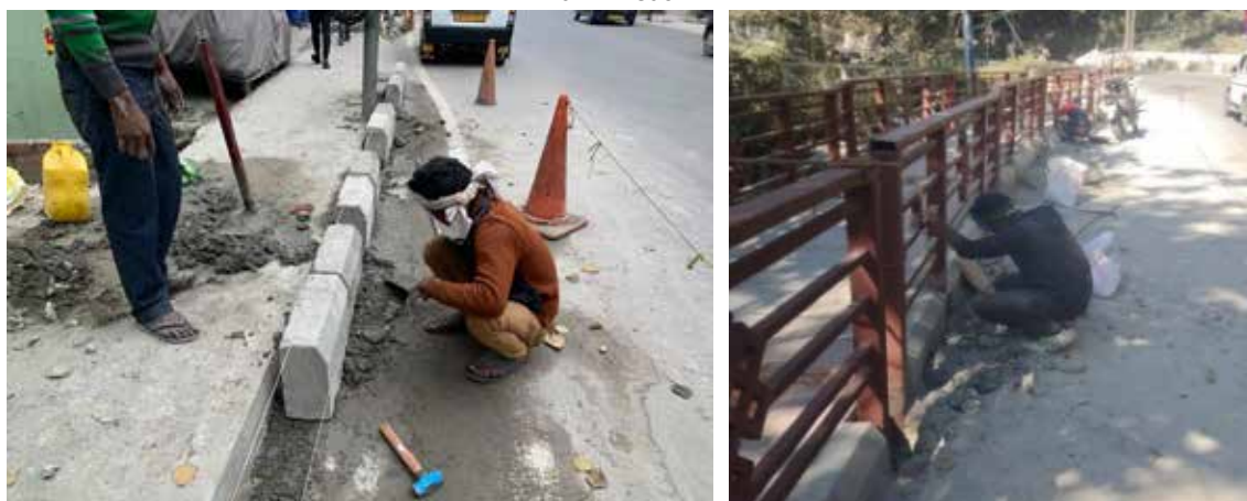
Figure 12: Laying of Kerbstones and Railings Source: GSCDL
