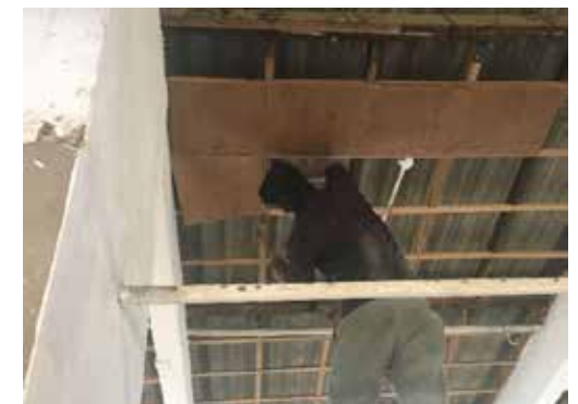
Figure 2.31: Process of fixing the jute sack ceiling, Source: Ar. Deepika Gandhi
