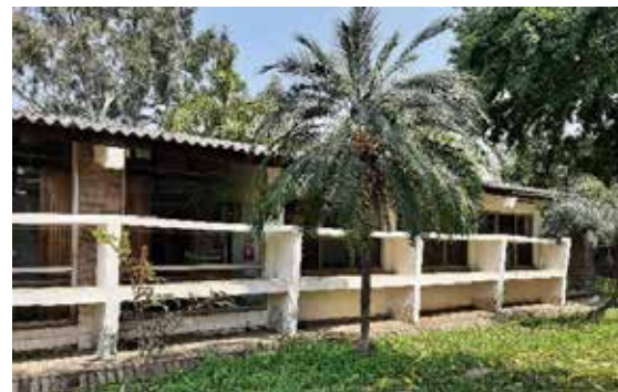
Figure 2.34 : Final restored louvres Source: Ar. Deepika Gandhi
